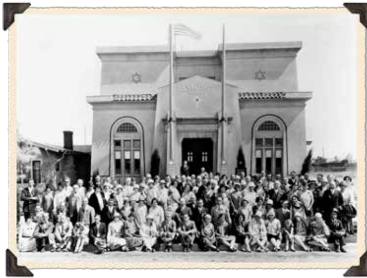
1928 Convention at Rosicrucian Park. Photo in front of the original Administration Building.
