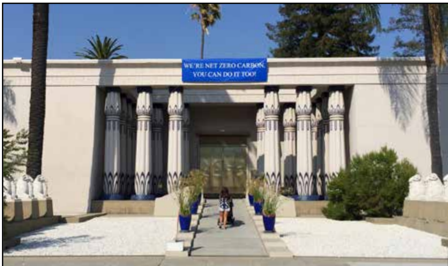
New wheelchair accessible entrance ramp to the Rosicrucian Egyptian Museum.
